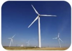
Electric Power Systems
